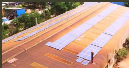
Hyderabad Factory installed with Solar Panels for Captive Power Generation
